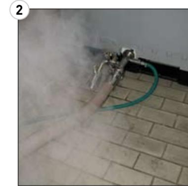
2 The outlet of the closed valve is steamed-sterilized prior to opening.
